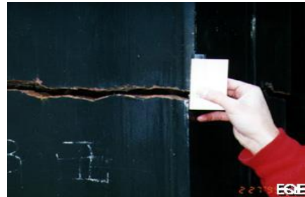
Figura 1.21 Columna fracturada transversalmente ( http://www.eqe.com/publications/kobe/building.htm )
